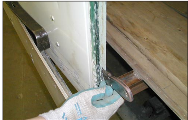
Illustration PL-65 Leveling Old Adhesive
