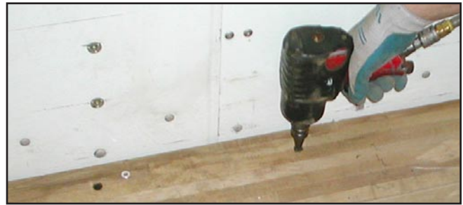
Illustration PL-45 Removing Floor Plank Fasteners
