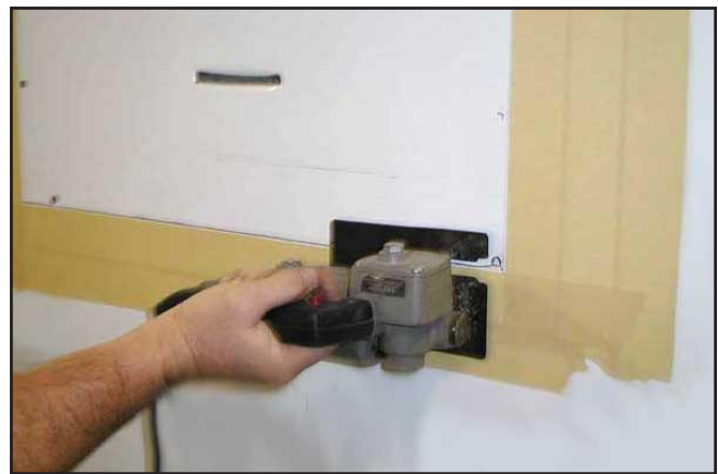
Illustration PL-25 Mark Off Damaged Area and Cut Out
