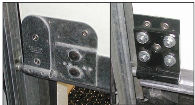
Illustration DR-55 Sample Bottom Roller Brackets
