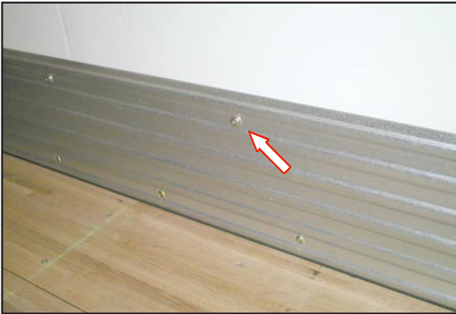
Illustration SC-5 Lower Scuff Plate (and Fasteners)
