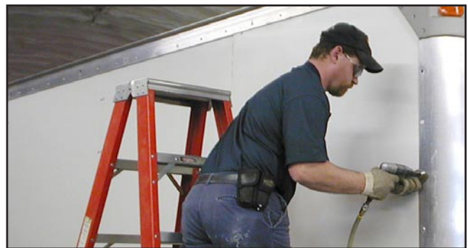
Illustration PL-55 Removing Panel Fasteners
