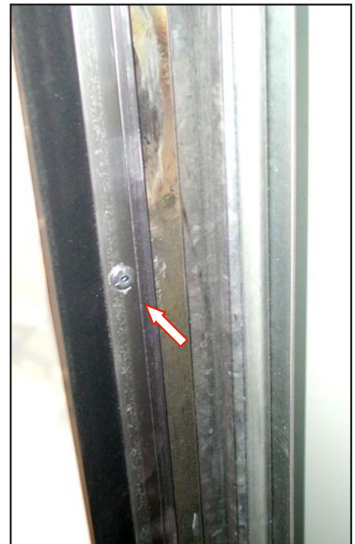
Illustration DR-90 Side Seal on Roll-Up Door
