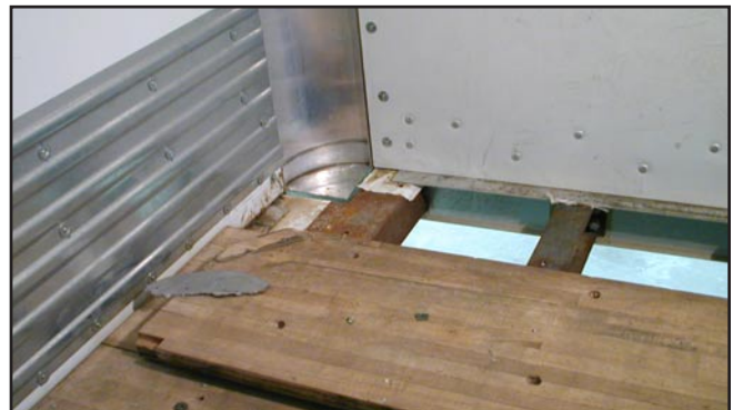
Illustration PL-50 Removing Floor Plank and Front Floor Cap
