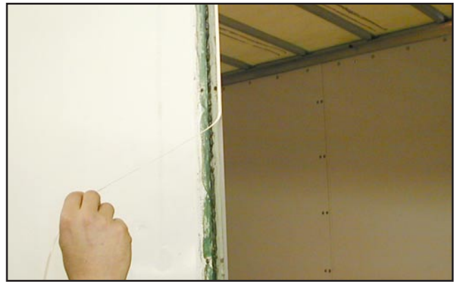
Illustration PL-75 Removing Tape Backing (Exterior Seam Side)
